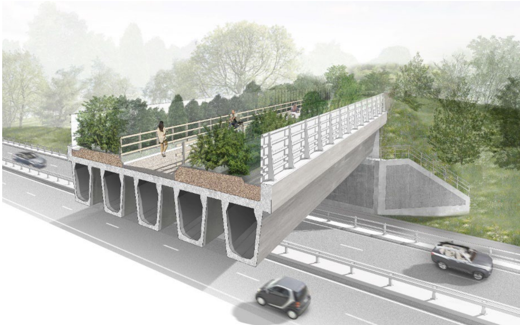
Figure 4-13 Illustrative typical cross section of a dual-purpose greenbridge structure with a central track
